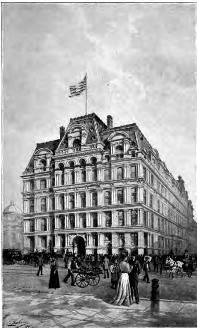
THE EQUITABLE BUILDING
